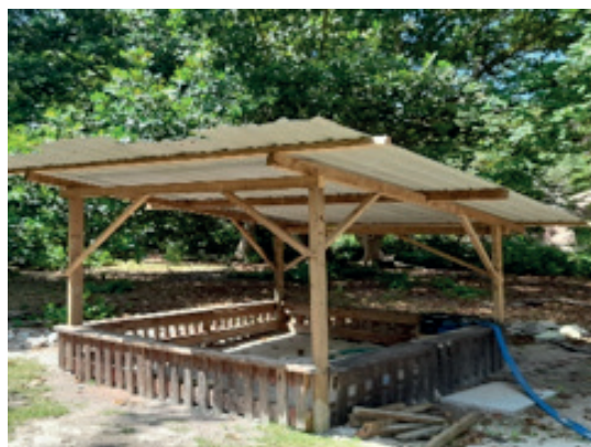
The new well
