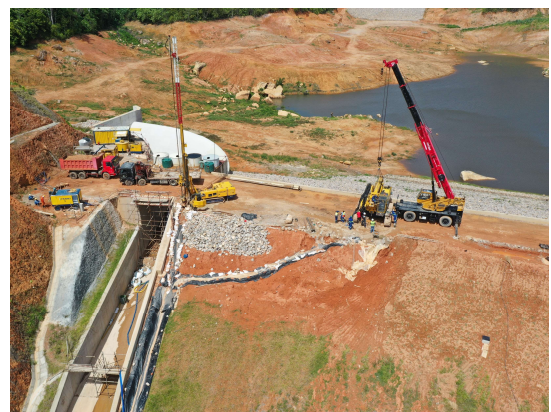
Embankment filling completed; Jet grouting works under spillway ongoing in September 2022
