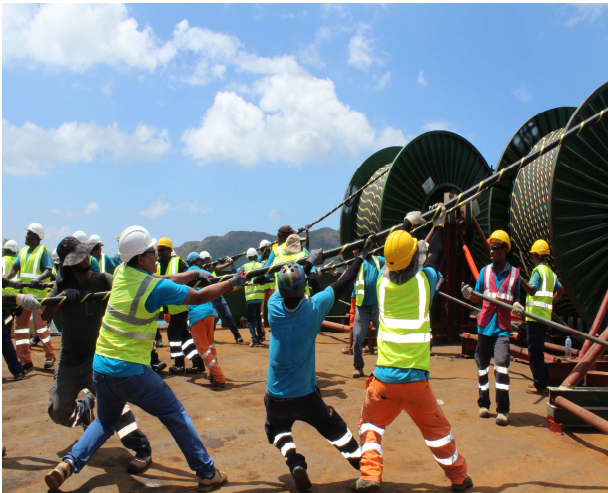
PUC team involved in cable laying operations
