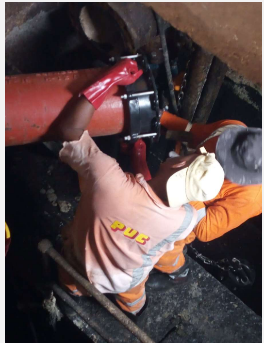
Wastewater team at work
