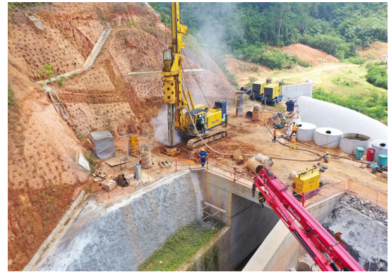
Piling works ongoing on right abutment in March 2022
