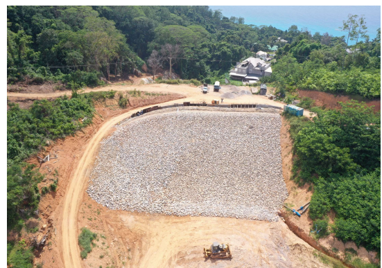
Construction of wave wall on south saddle dam ongoing in March 2022
